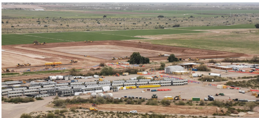
Laydown area at Florence Copper (foreground) site preparation (background)
